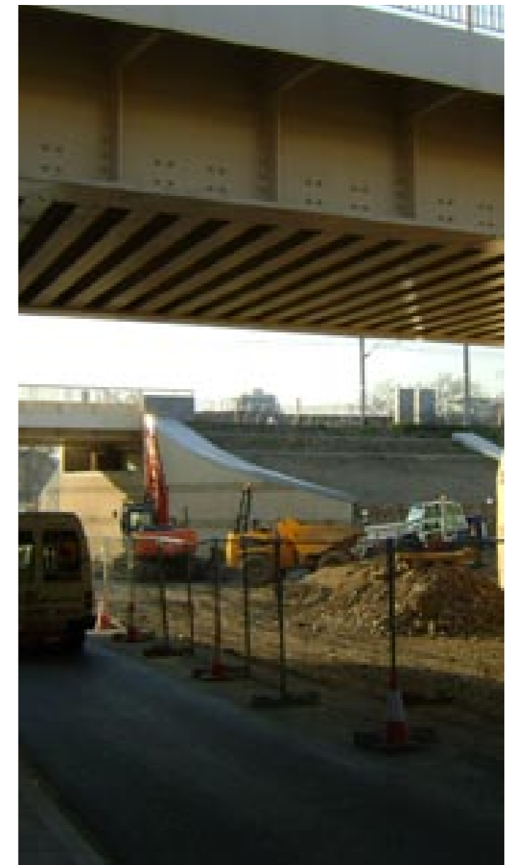
The new Aerodrome Road bridges being constructed
