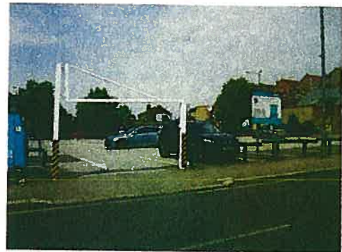
Perryfield Way car park
