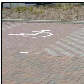
**Figure C.3 - Illustration of a Pervious Pavement using Block Paving**
