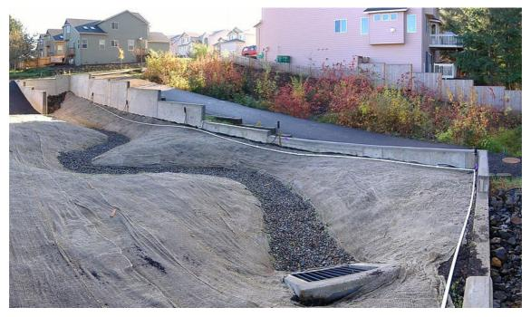
Figure E2-7 Example of swale under construction (completed swale shown in background)
