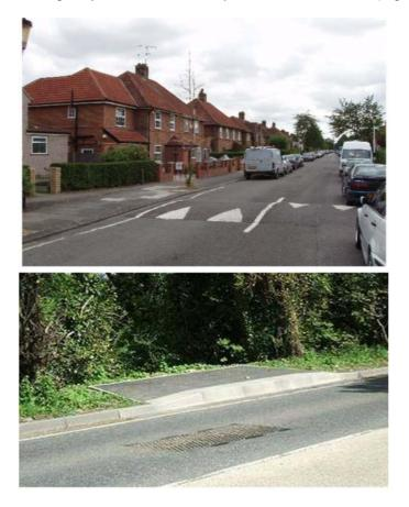
Figure E2-11 Example of a speed hump (Geograph, 2011<sup>ix</sup>) and of raised kerbing (Barkingside, 2009<sup>x</sup>)
