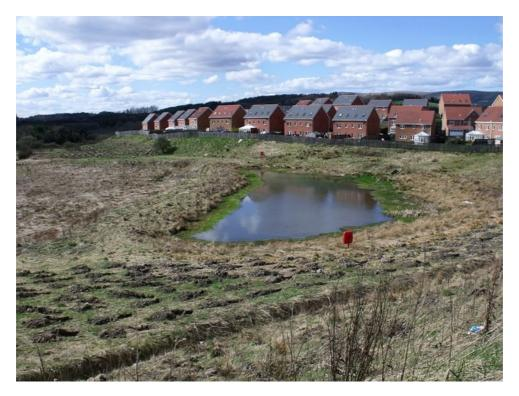
Figure E2-8 Example of Detention Basin  $\ensuremath{\textcircled{O}}$  Copyright BJ Smur^{vi}
