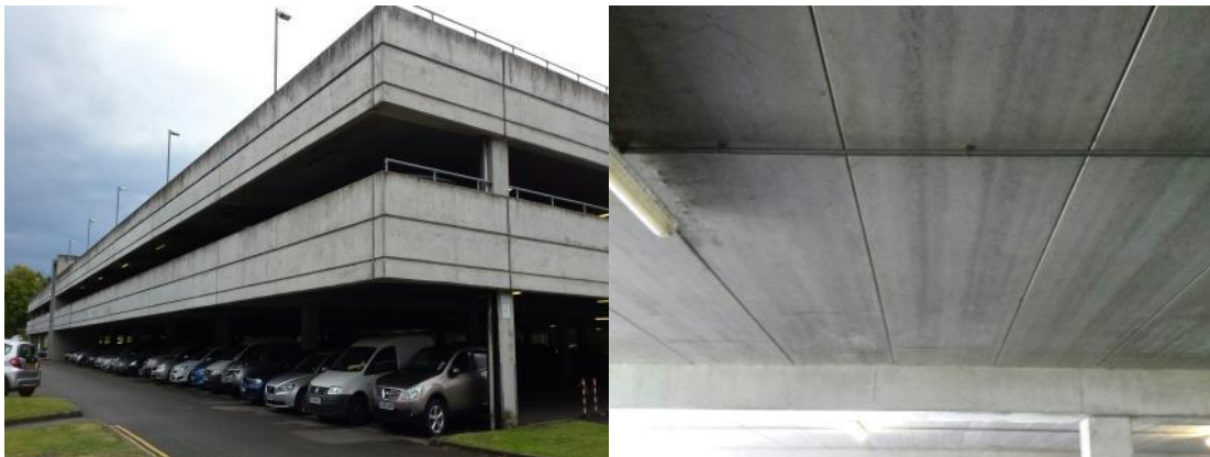
Photograph 20 & 21. Building B10 car park
