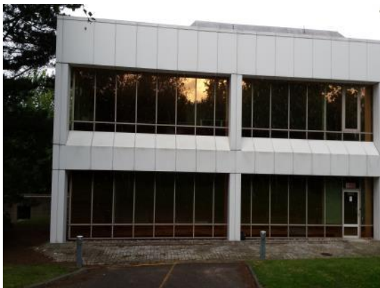
Photograph 19. External features of building B9
