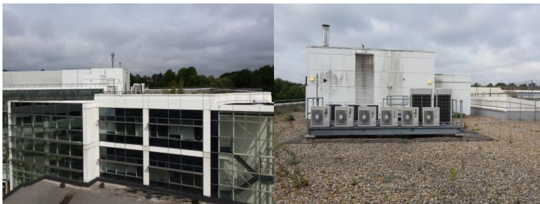
Photographs 6 & 7. Photo 6 (left) shows building B1b from B1a, both have the same construction. Photo 7 (right) shows the roof of B1a, which is similar to B1b.
