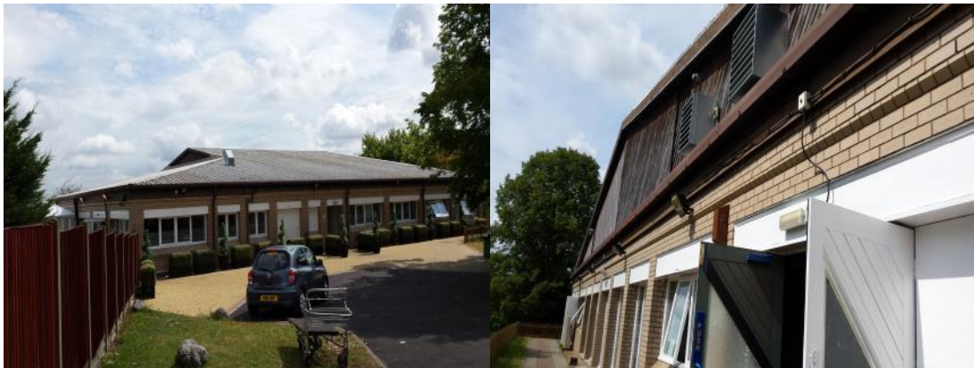
Photograph 11 & 12. Building B3 external features
