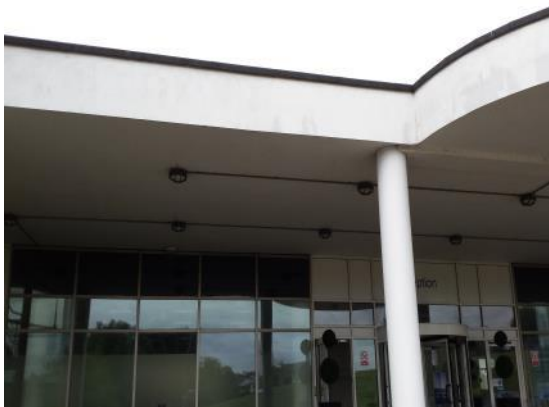
Photograph 10. Single storey flat roofed reception of building B1g
