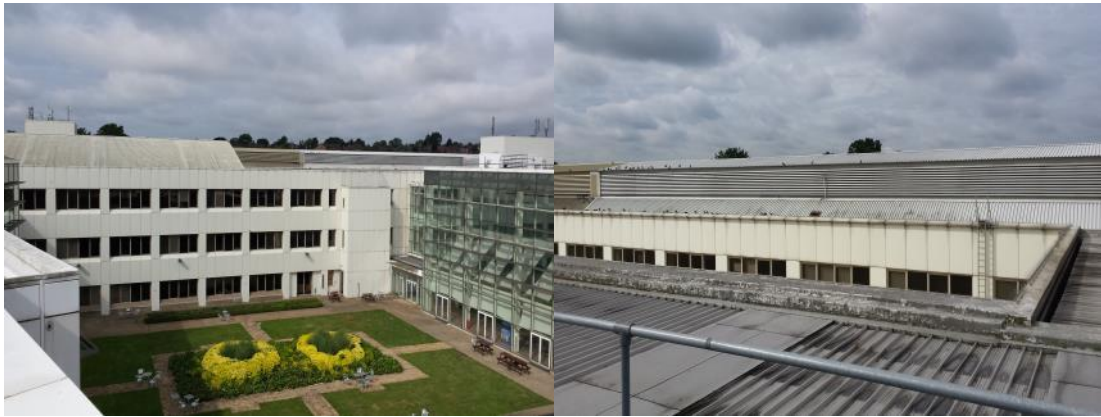
Photographs 8 & 9. Photo 8 (left) shows B1c from B1a. Photo 9 (right) shows the roof of B1c and the joining roof of B1d.
