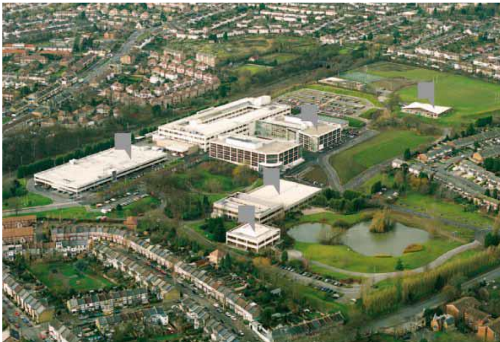
Fig. 1: Aerial view of the site from the south east (from DAS p6)
